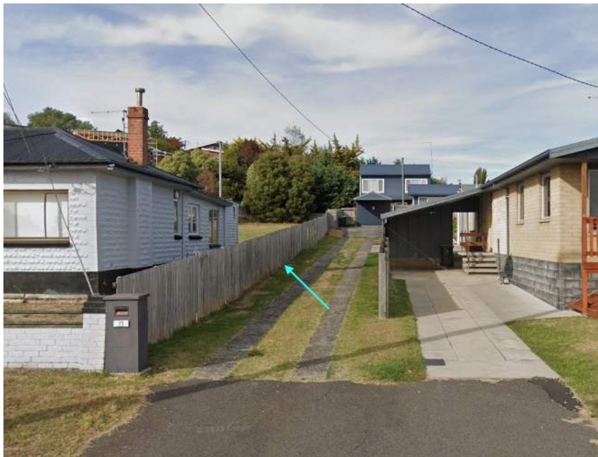
Figure 2 – Street view of the access to 17 and 17A Alice Street and location of the proposed retaining wall
