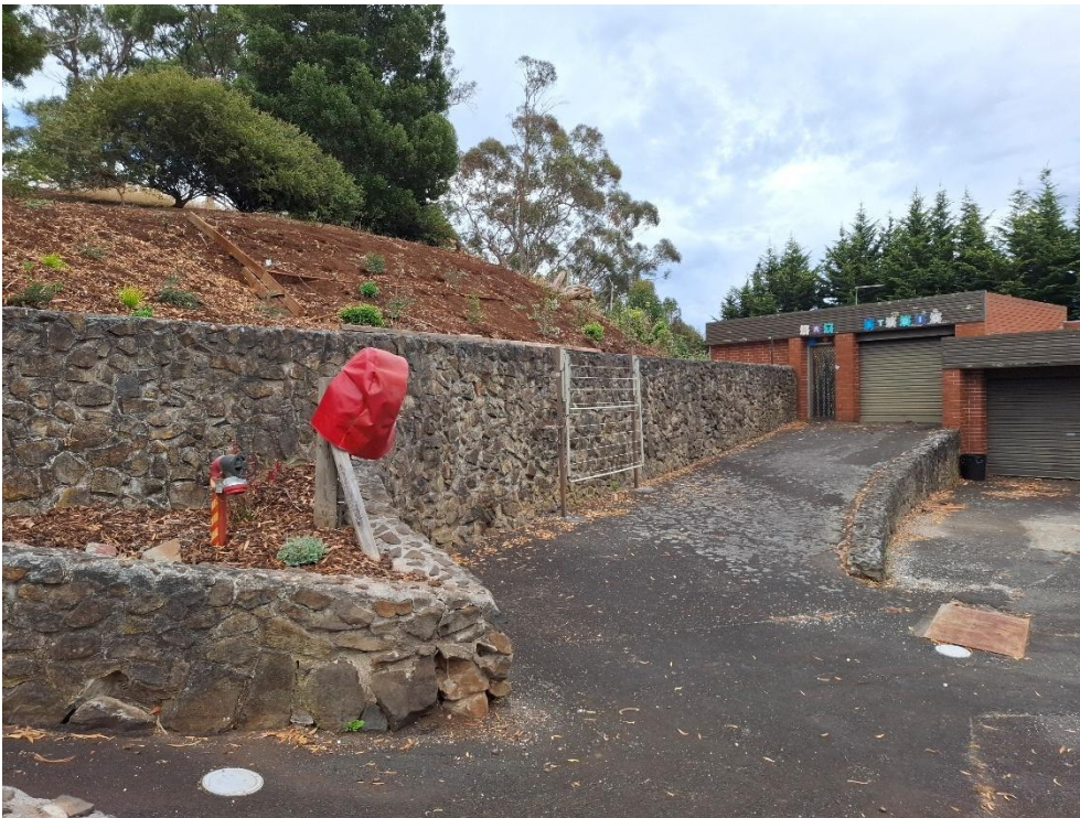
Image 5.1.1- Existing internal hydrant
