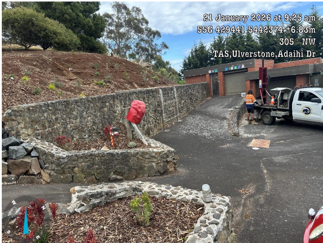
Plate 1 – View of the proposed extension area and existing retaining walls, 21.01.2026
