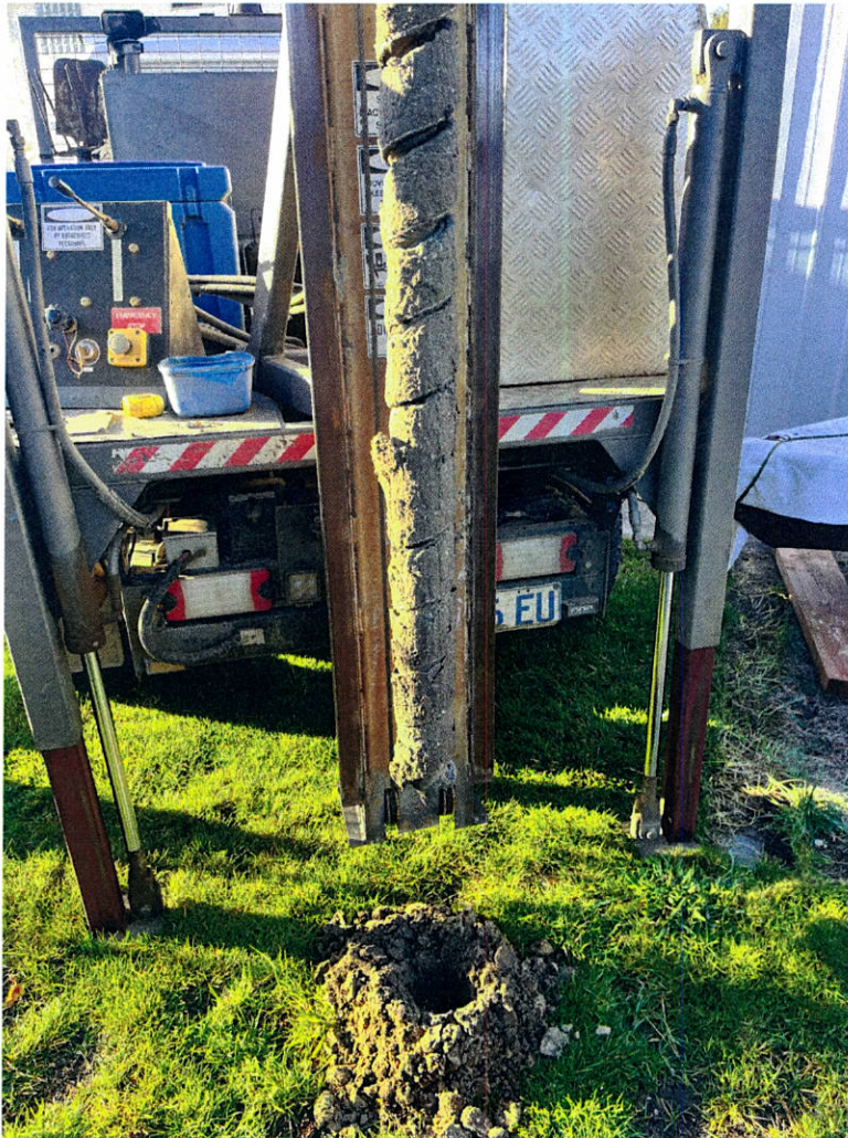
Plate 3 – Test Hole #1- looking to the southeast.
