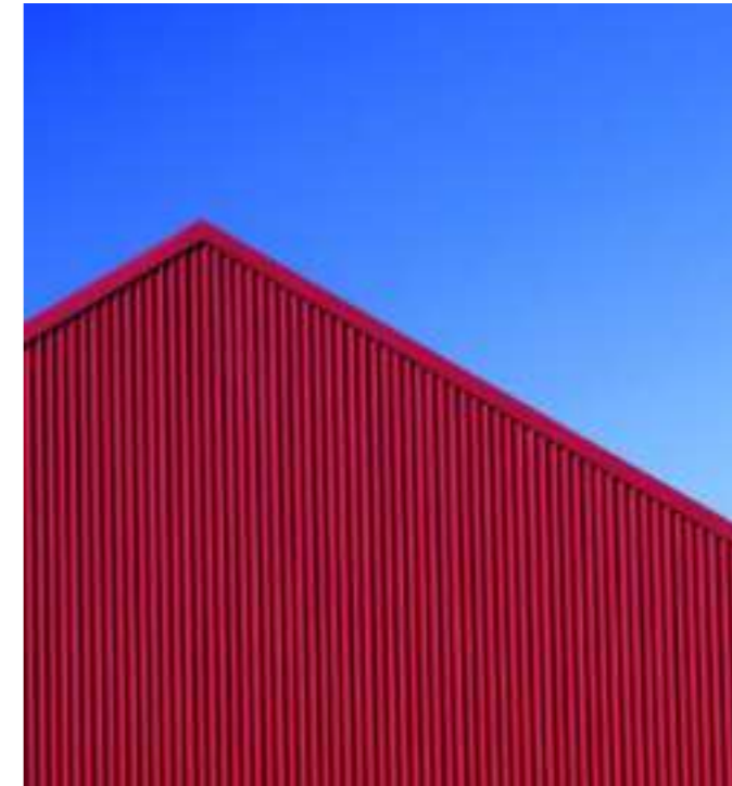
03 MANOR RED CORRUGATED METAL FACADE CLADDING, FLASHING, CAPPINGS, METAL DOWNPIPES, GUTTERING & ROOFING
