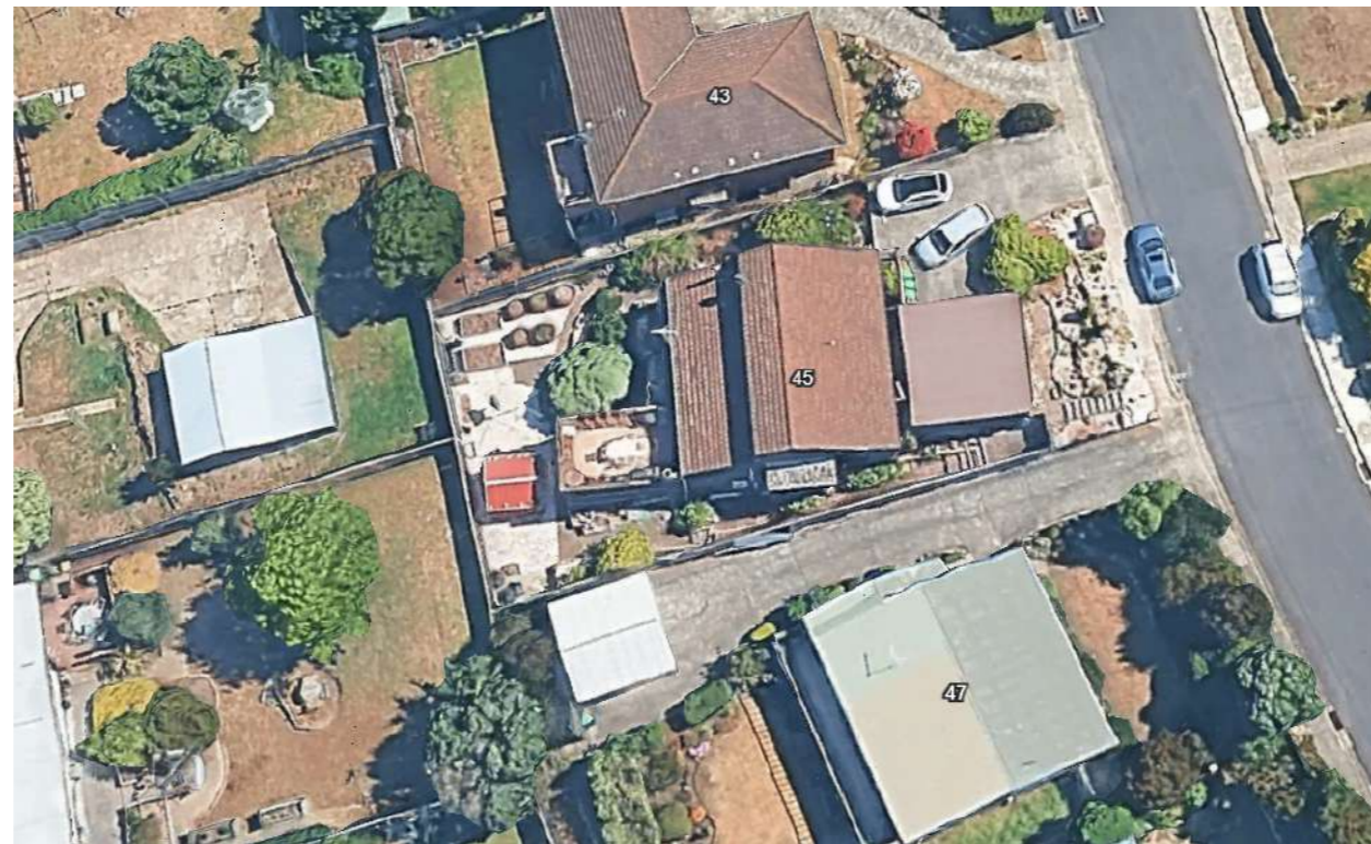
THE ADJACENT PROPERTY LOCATED TO THE SOUTH-EAST OF SUBJECT SITE HAS VEHICULAR ACCESS/ CONCRETE DRIVEWAY BESIDE THE EXISTING LAUNDRY, WITH THEIR PRIVATE OPEN SPACE LOCATED SOME DISTANCE AWAY FROM THE PROPERTY BOUNDARY.
