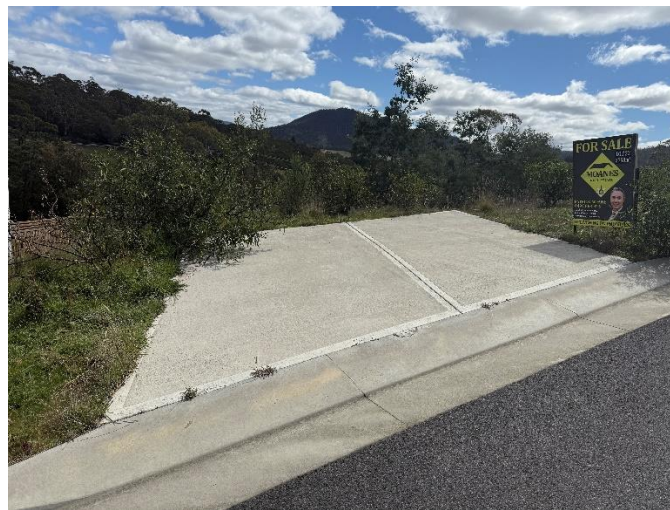
Figure 5 – Existing concrete apron into Lot 5
