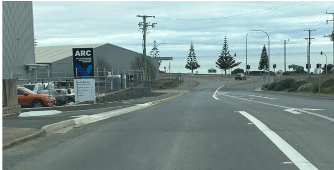
Figure 7 – Massy - Greene Drive Southern approach to development site.
