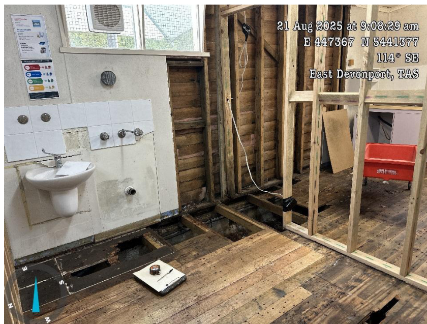
Plate 2 – View of Borehole BH2 location inside the early learning building, 21.08.2025
