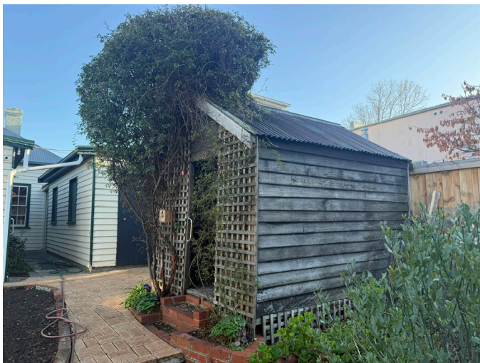
Figure 10: Timber outbuilding (Source: Purcell)
