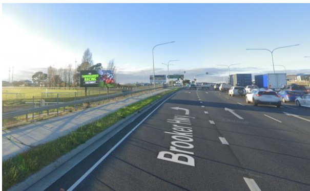
Figure 2: Sign located on Brooker Highway at Elwick Racecourse
