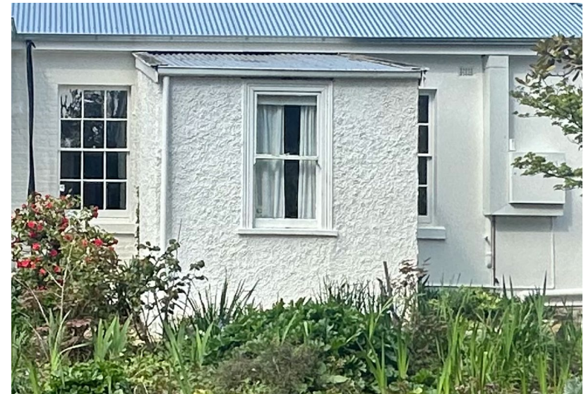
Contrasting wall treatments on the western elevation – face brick, textured stucco and render.
