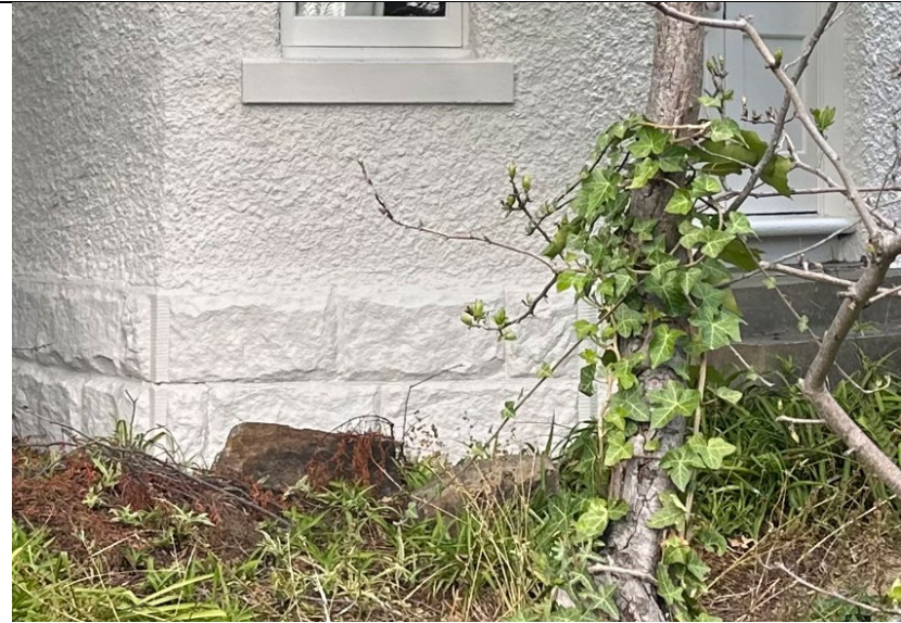
Example of textured stucco on the 1920s addition. Note the rusticated sandstone foundations.
