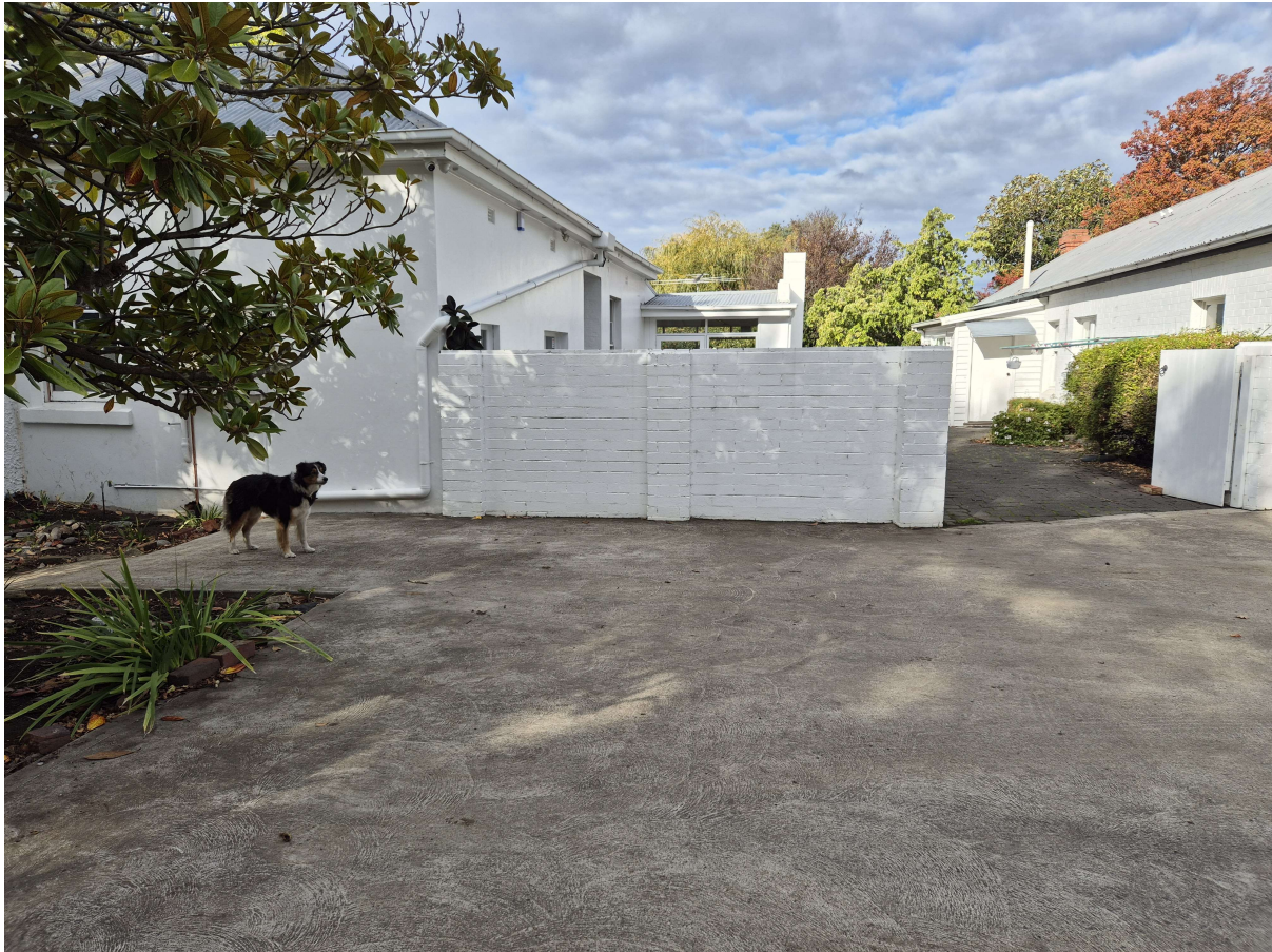
Image 8. The brick courtyard fence where it meets the existing dwelling. Refer to demolition plan for the location of image 8.
