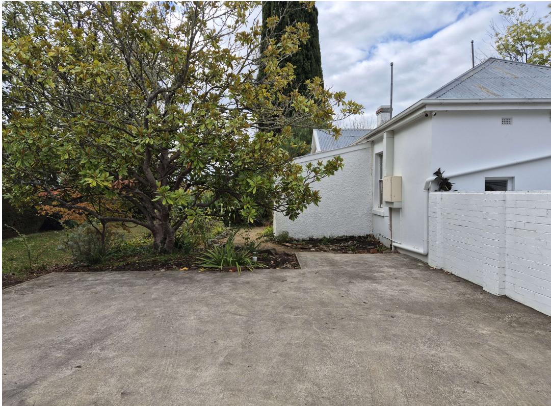
Image 1: Lean to A viewed from the rear of the building. Refer to Demolition plan for the location of image 1
