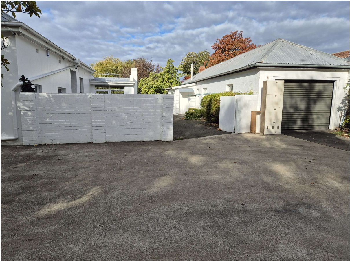
Image 7. The class 10 building south western facade showing the garage roller door and brick courtyard fence. Refer to demolition plan for the location of image 7.
