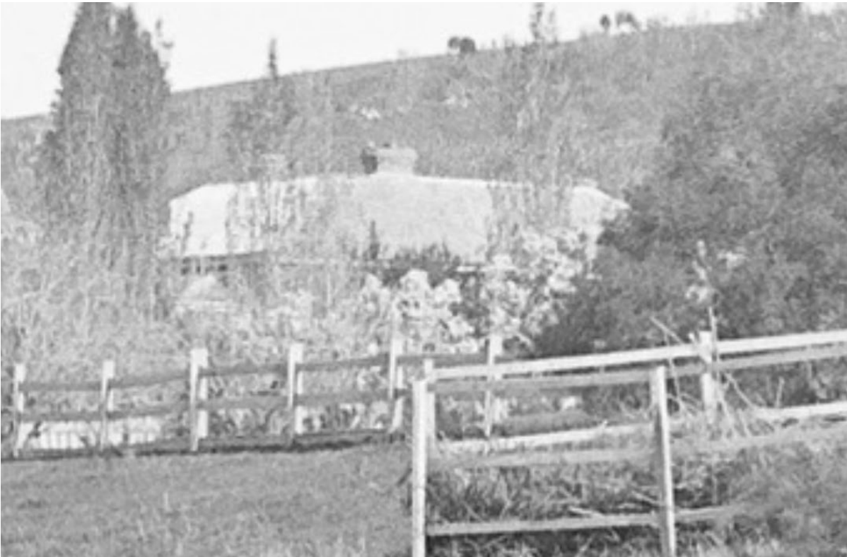
This photograph shows the roof form and chimneys, and some landscape elements of The Elms.
