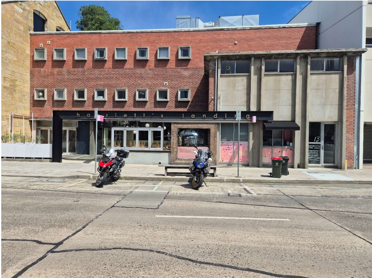
Image 03 Existing Castray Esplanade facing façade. Image Supplied Room 11 Architects 27/11/2025.
