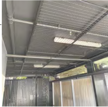
IMAGE 01. EXISTING FLUORESCENT LIGHTS IN FRONT OF CAFE/RESTAURANT.
