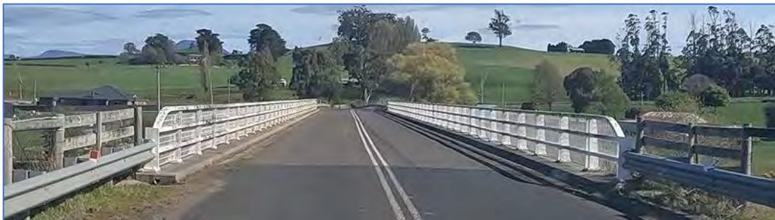
Photograph 5.2C – Bridge over the Bass Highway
