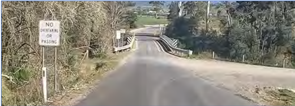
Photograph 5.2B – One Lane bridge over the Meander River
