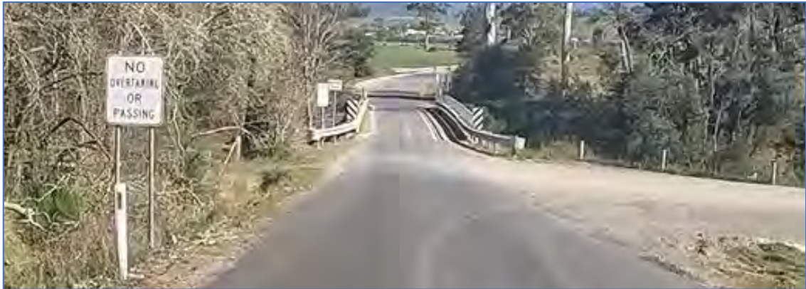
Photograph 5.2B – One Lane bridge over the Meander River
