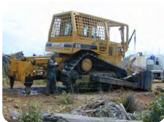
Portable vehicle washdown unit is used to provide water with disinfectant. Note any surplus water present in the tank should be drained to limit the amount of disinfectant released into the environment. Photo courtesy of Forestry Tasmania.
