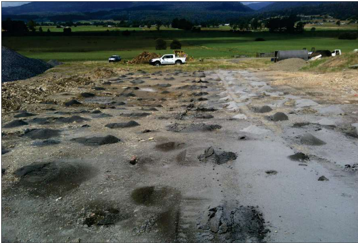
PLATE 9 - Blast drill pattern to the south of the existing quarry
