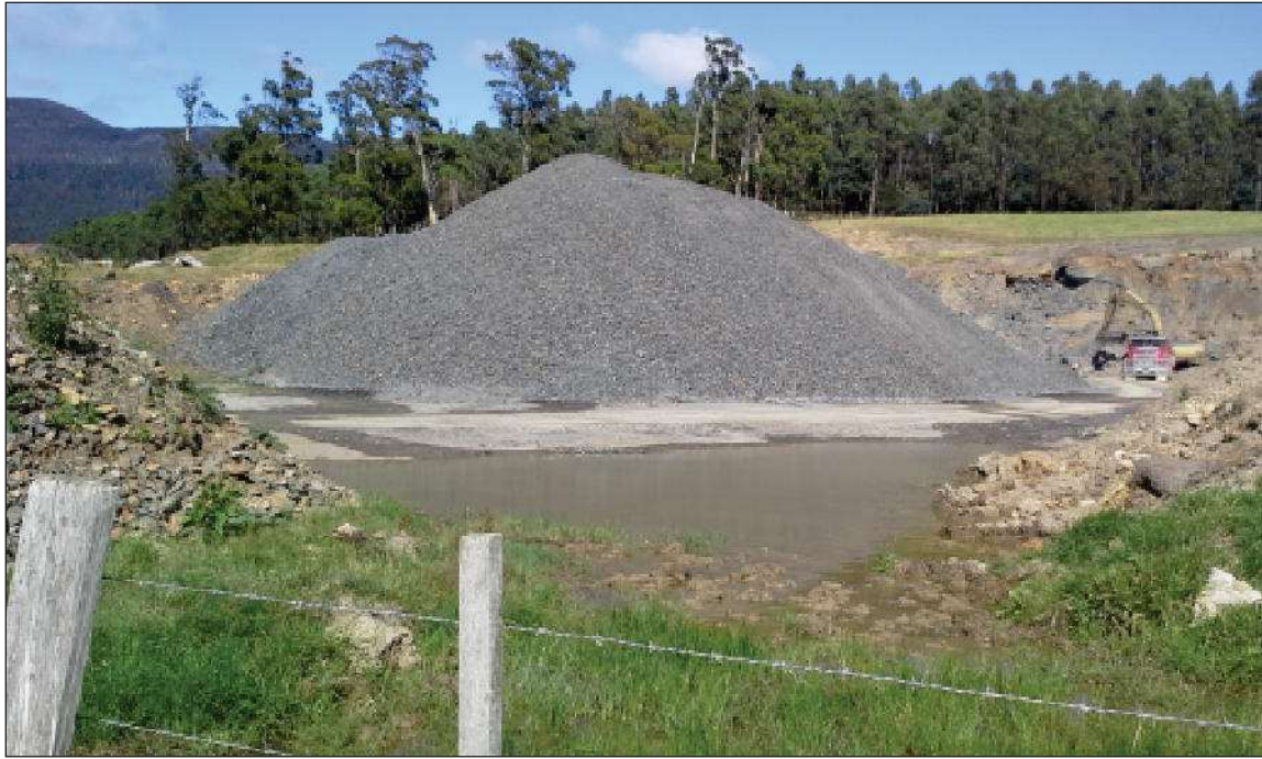
PLATE 13 - View of sediment basin to the west
