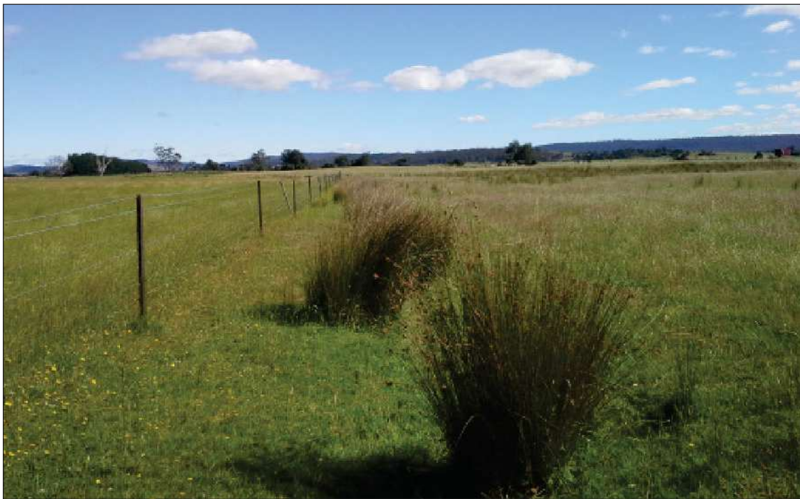
PLATE 14 - View of the vegetated drainage channel looking north
