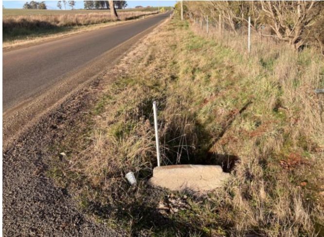
Figure 10 – Side view of access to 1303 Osmaston Road
