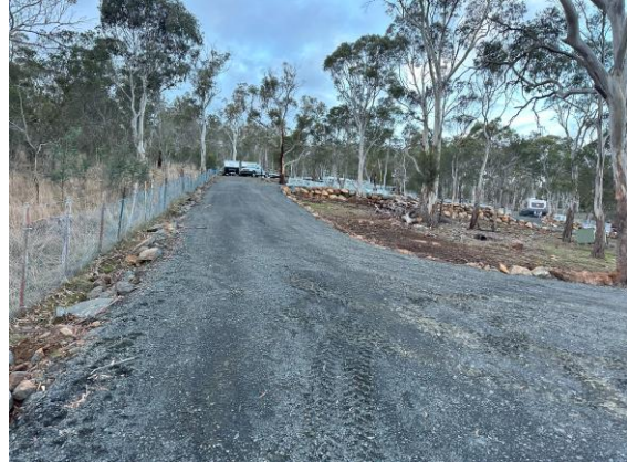
Driveway also continues to top section of access
