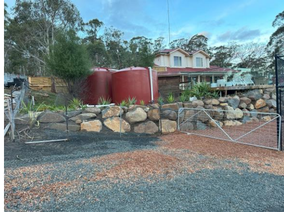
Hardstand area is close to the tank, however a remote offtake may be required to ensure ease of use and access by firefighting personnel
