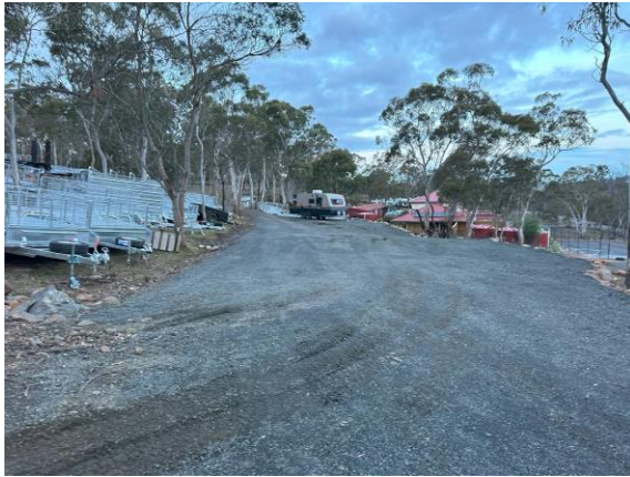
Top section of driveway
