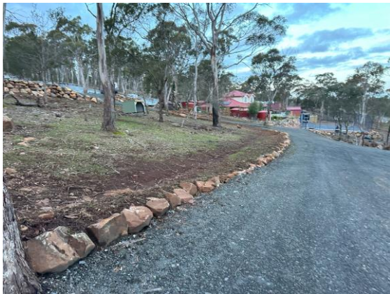
Bottom section of circular driveway
