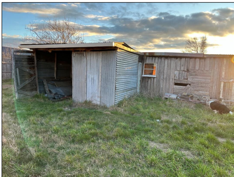
Figure 1: View of the large outbuilding on Lot 2 from the East
