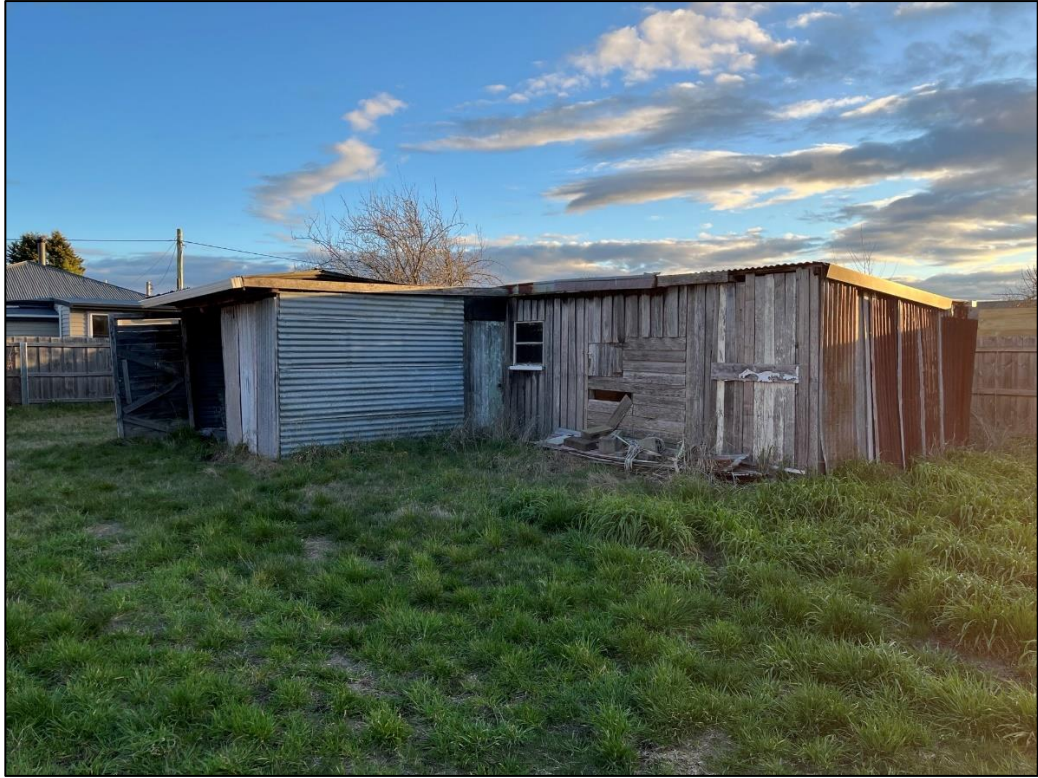
Figure 2 : View of the large outbuilding on Lot 2 from the North
