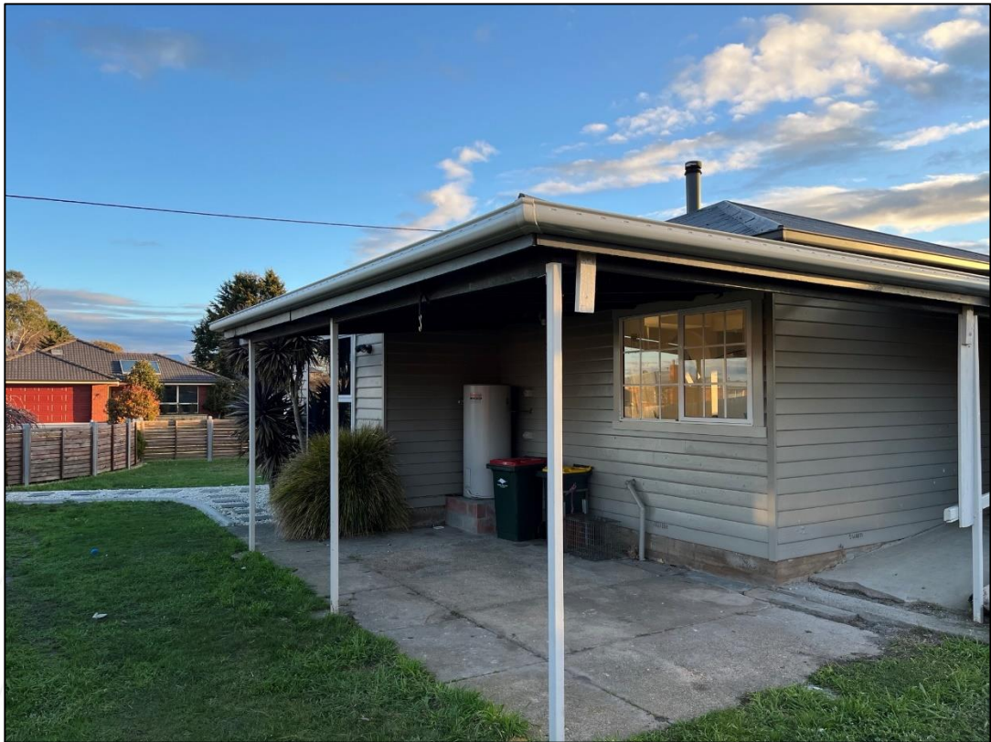
Figure 4: View of the verandah from the northeast of the dwelling
