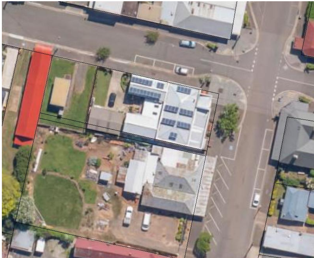
Figure 3 – Aerial view of 14B Lyall Street, Westbury
