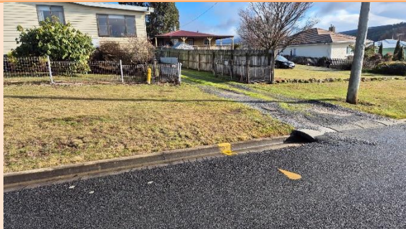
Existing hydrant in Caveside Road (Lot 3)
