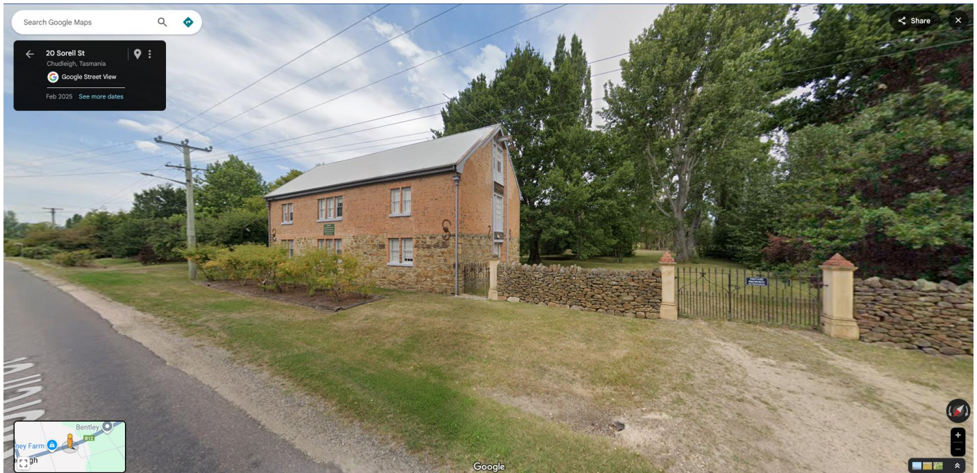
Figure 5: Lot 1 building (Google Street view)
