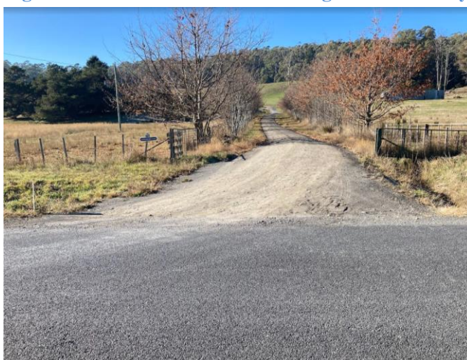
Figure 15 – Elevation view of existing Lot 1 driveway from Huntsman Road.
