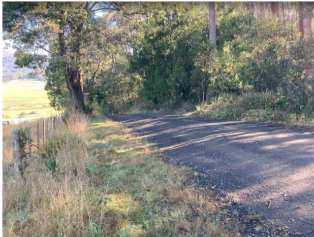
Figure 29 – Looking left along Sherriffs Road from proposed access to Lot 2.
