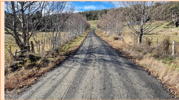
Existing access and driveway (approx. 4.1m wide) – Lot 1
