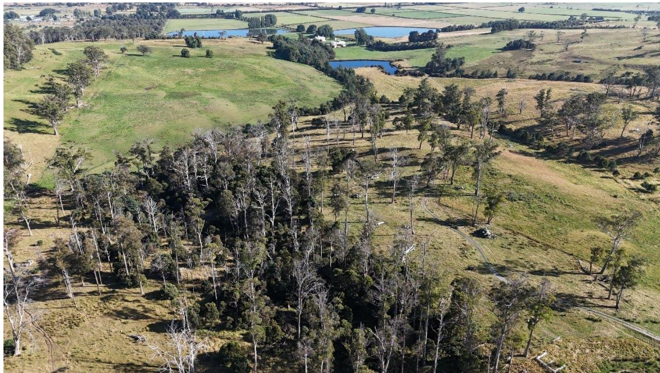
Image 16 Aerial image taken from the south west area of the property looking north, with Bentley house and the land subject to the development visible in the centre of the image. (taken on the site assessment 21/1/2025)
