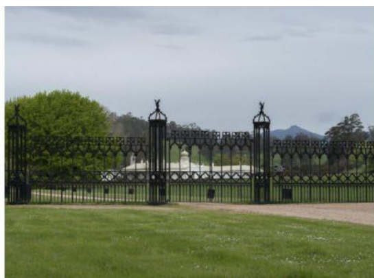
Plate 2. View to formal gates
