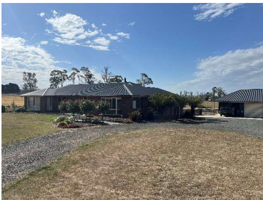
Figure 10 The existing dwelling in lot 1.
