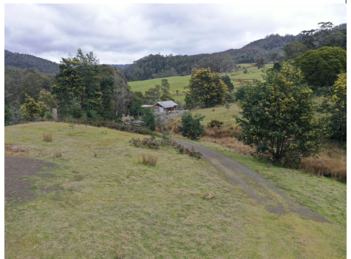
Driveway ends level with building site. Drainage is excellent and soil has proved stable for heavy trucks (35t) even in the wet.
