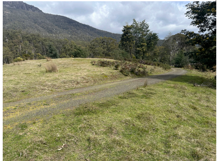
Existing rolled road base driveway - this access has existed on the property for many years with no erosion
