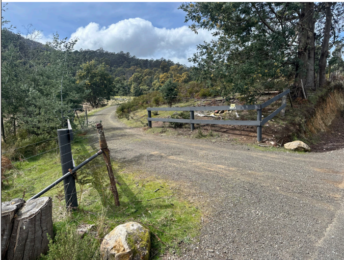
Existing driveway - Looking back to the gate
