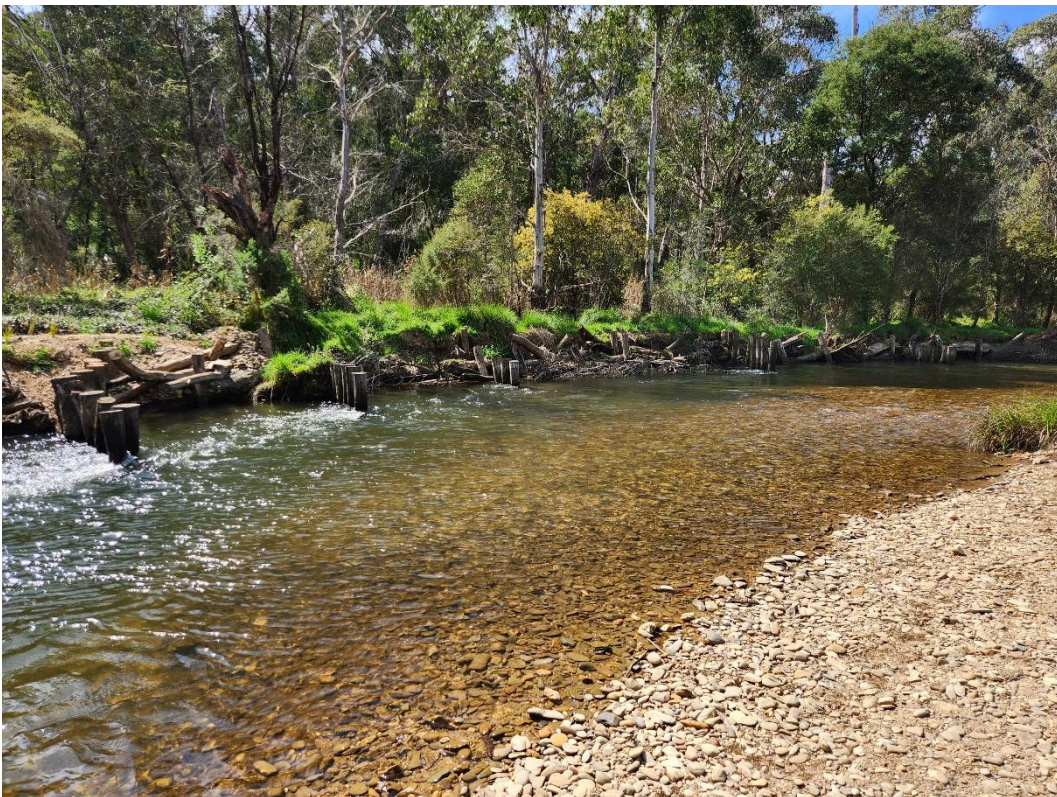
Figure 2-3 Timber revetment and pile fields within a cobble bed river.
