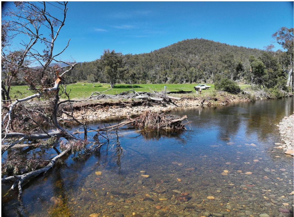
Figure 3-3 Looking across at a section of bank erosion on the southern floodplain.
