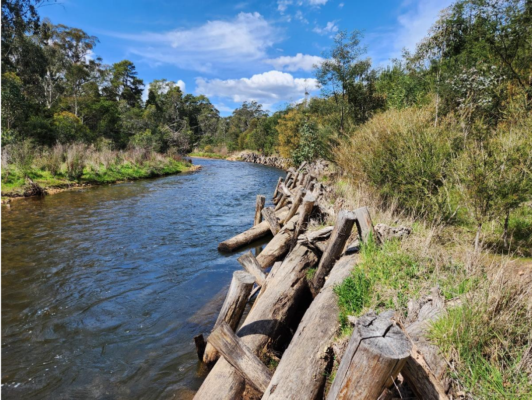
Figure 2-2 Timber revetment and revegetation.
