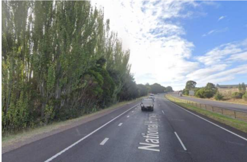
Figure 32 –East bound carriageway of the Bass Highway adjacent 90 Trevor St.
