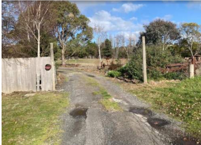
Figure 10 – Looking left along Walker Street from Trevor Street
