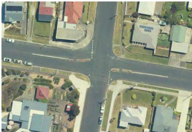
Figure 13 – Aerial view of Leven / Walker Street intersection
