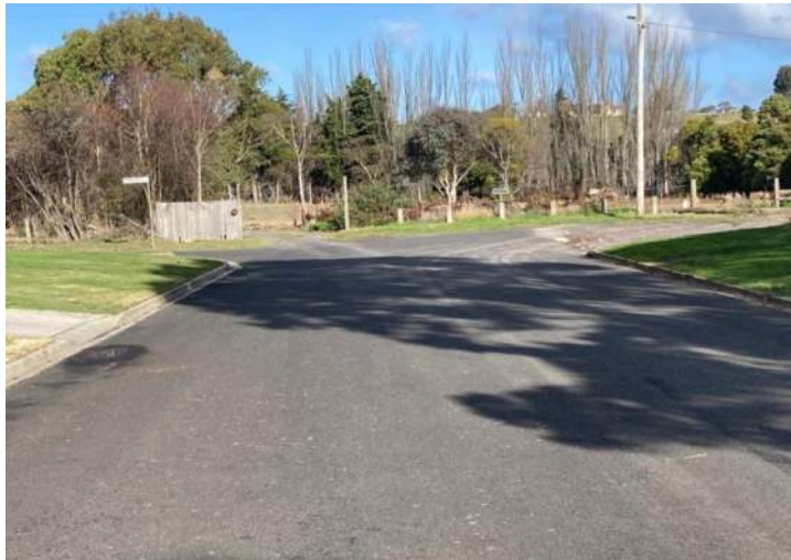
Figure 8 – Trevor Street approach to Walker Street
