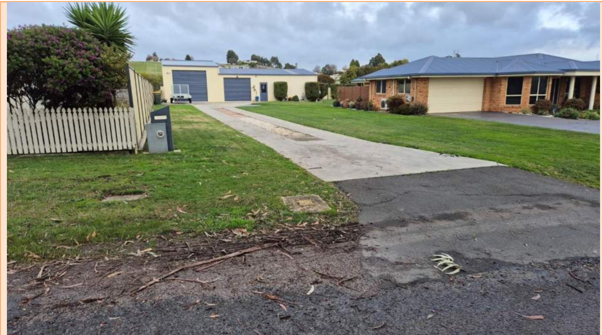
Existing fire plug – adjacent to 78 and 80 Trevor Street
