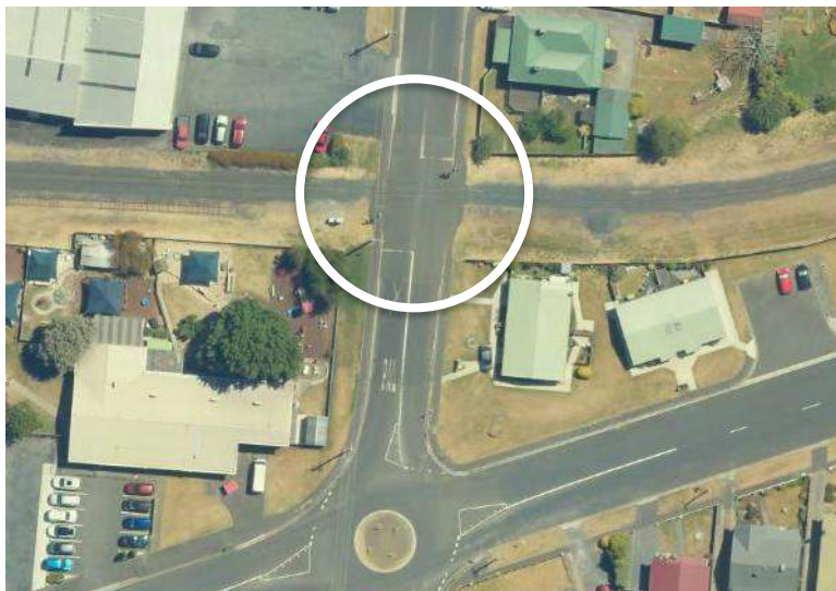
Figure 21 – Aerial view of the James Street Level Crossing
