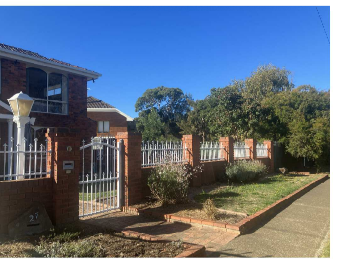
EXISTING FRONT FENCE BEING REPLACED
