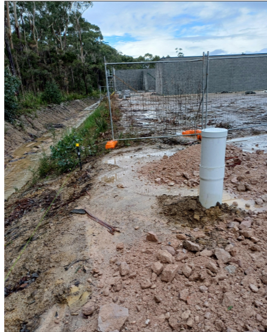
LOOKING EAST AT REAR NORTH EAST CORNER OF BLOCK
