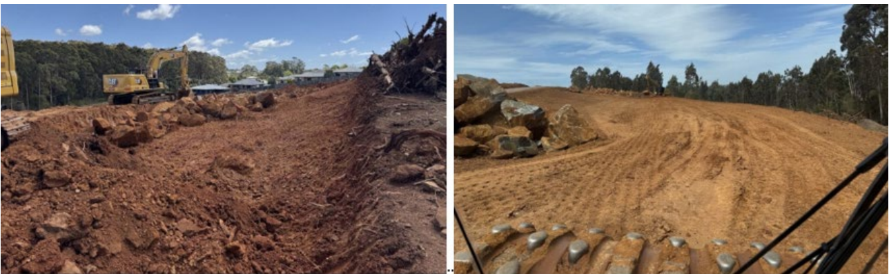
Figure 1 - Photographs approved lot levelling lots 3-11; spoil used to fill lots 15-21
