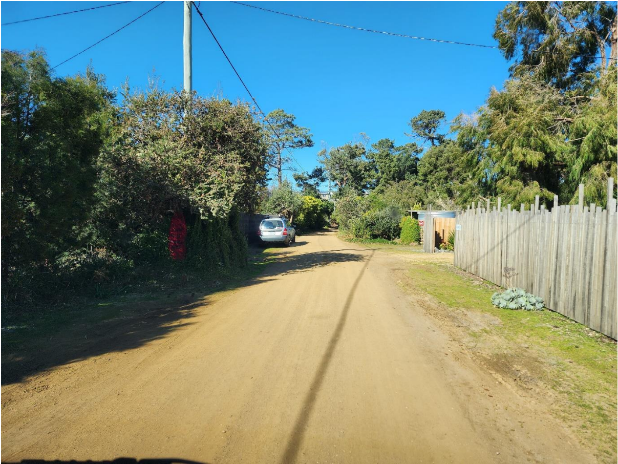
Looking Southeast along Thompson Way
