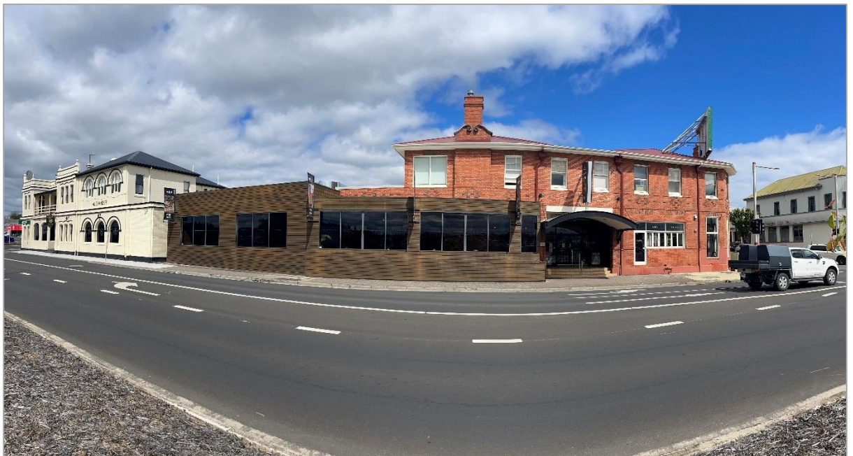
Figure 2 Site photo, from Formby Road. Development area proposed in centre of image, set back from the road and frontage, adjoining the second storey
