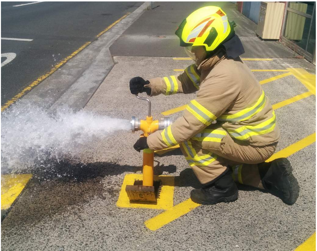
Figure 9 A firefighter accessing water from a ground ball hydrant via standpipe connection
