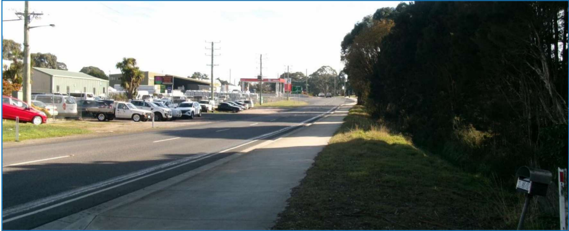
Photograph 7.2A – Available sight distance to the right
