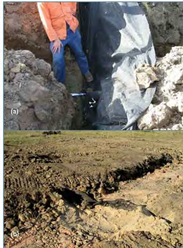
Figure 15. (a) Installation of sandblock perpendicular to a service trench. Note securing of geotextile to the optical fibre cable to prevent water flowing past the sand block. (b) Sandblock before final topsoiling.
