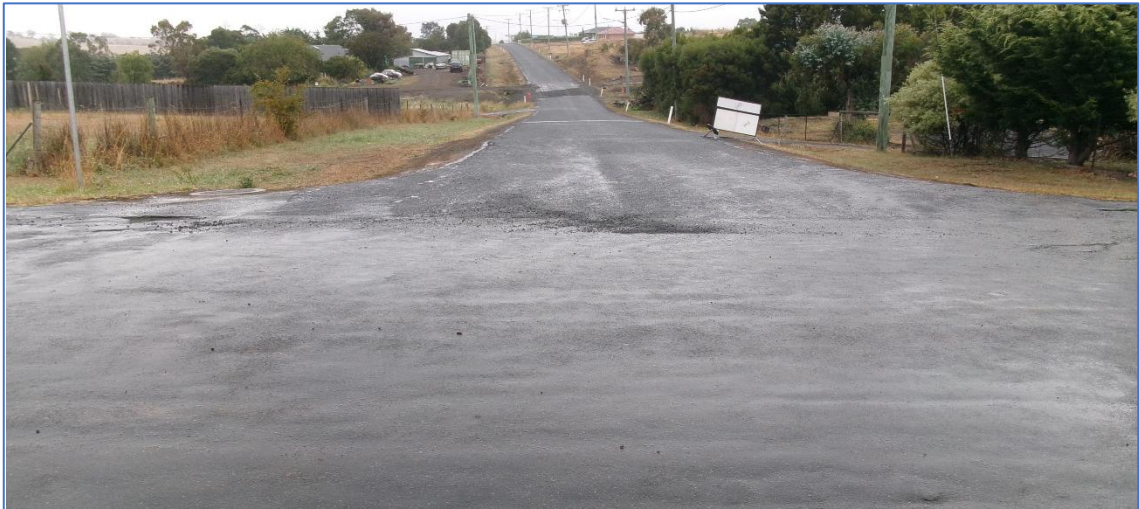
Photograph 5.3 – Dylan Street and William Street junction
