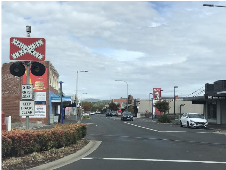
Figure 10 – Reibey Street Eastern approach at Level Crossing
