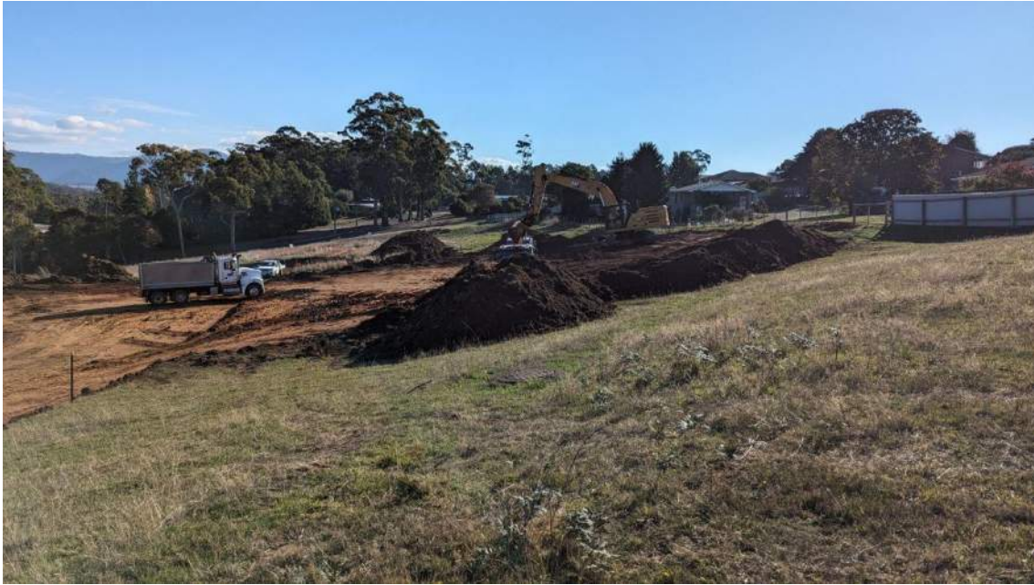
Plate 1: View of the proposed excavation area looking to the west
