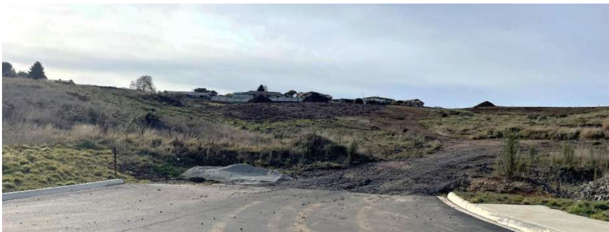
Figure 3 - Site photo, facing north and east, June 2024
