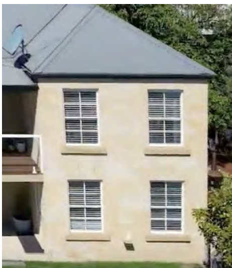
The exiting dwelling with sandstone masonry walls, grey roof and white double hung multi-pane windows
