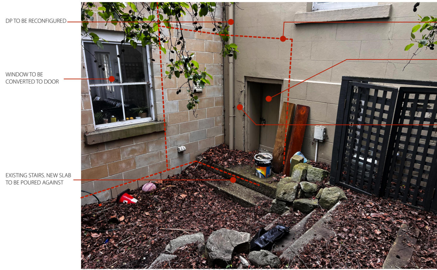
EXISTING SITE CONDITION SWITH PROPOSED WORKS OVERLAID
