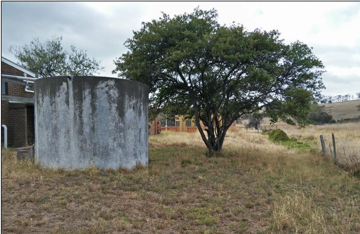
Photo 6 – Existing water tank on proposed Lot 7 (33 Spitfarm Road)
