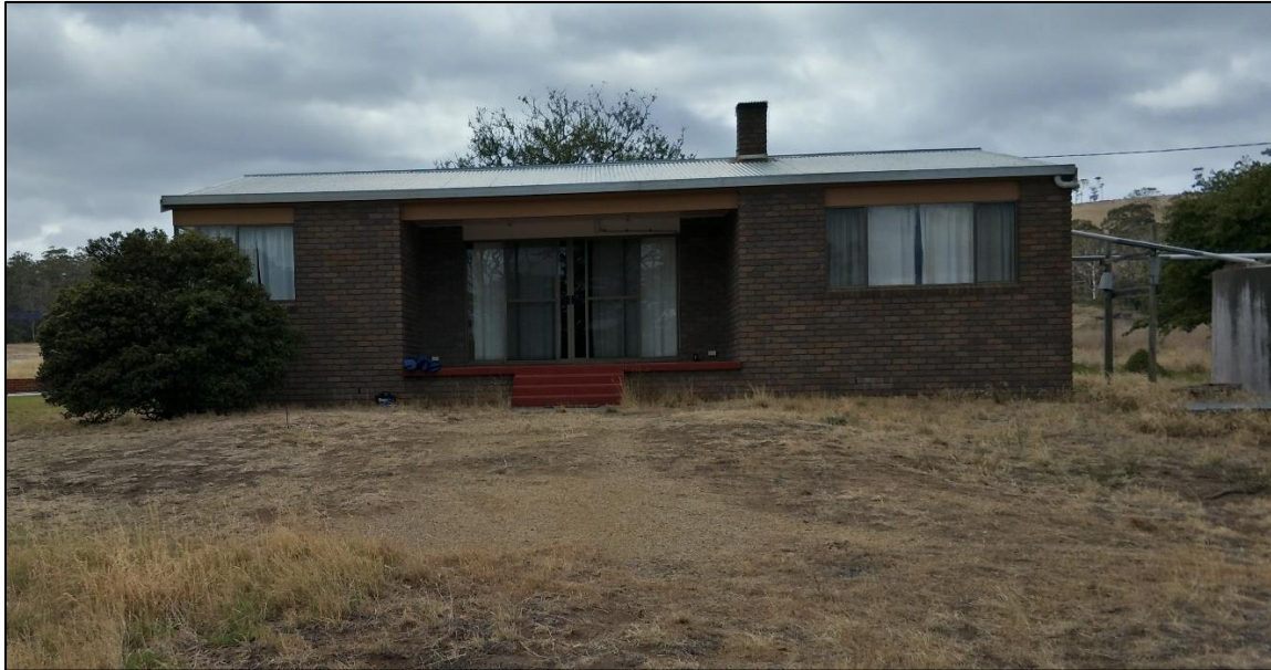
Photo 5 – Existing brick one-storey dwelling on proposed Lot 7 (33 Spitfarm Road)
