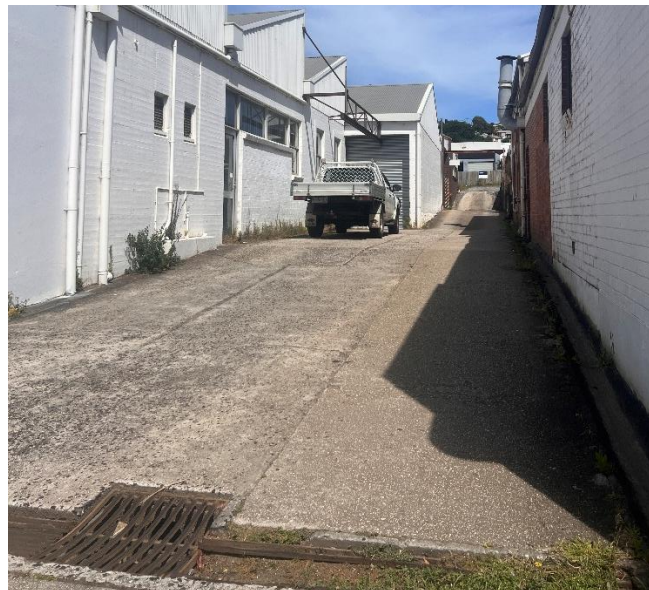
Figure 8: Existing Site Access Laneway from Wilson Street
