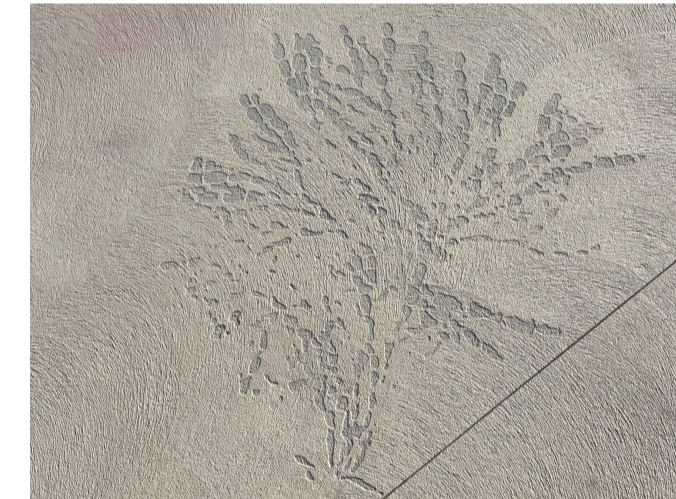
Image 01: HS03 - concrete sandblasting
