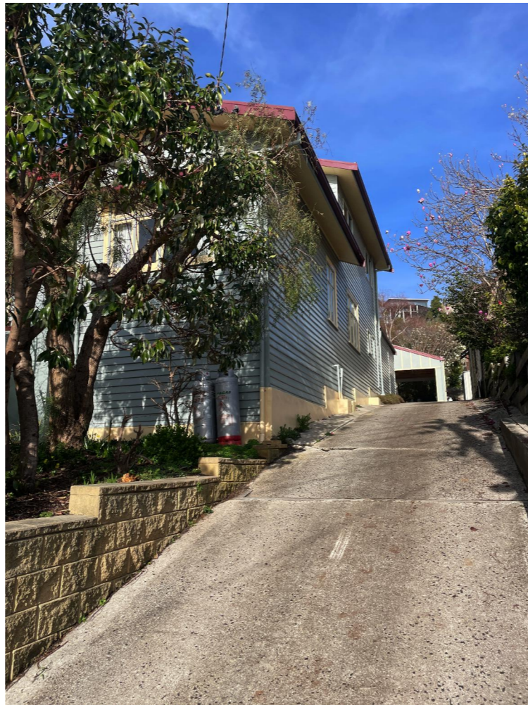
VIEW OF WEST FACADE FROM FRONT
