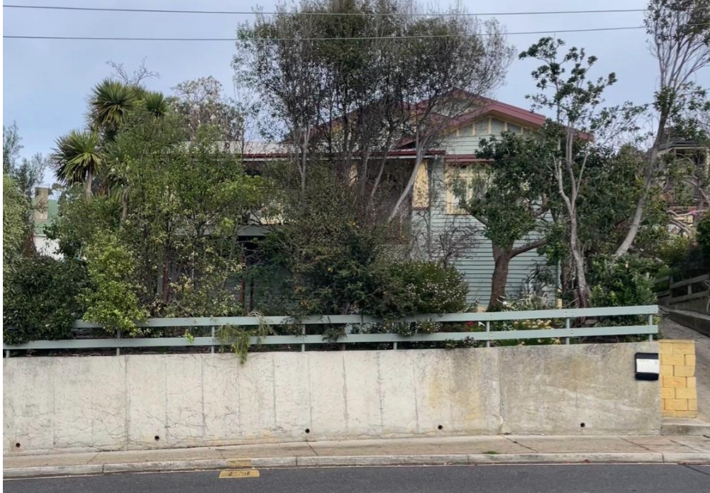
VIEW OF NORTH FACADE FROM OLIVE STREET
