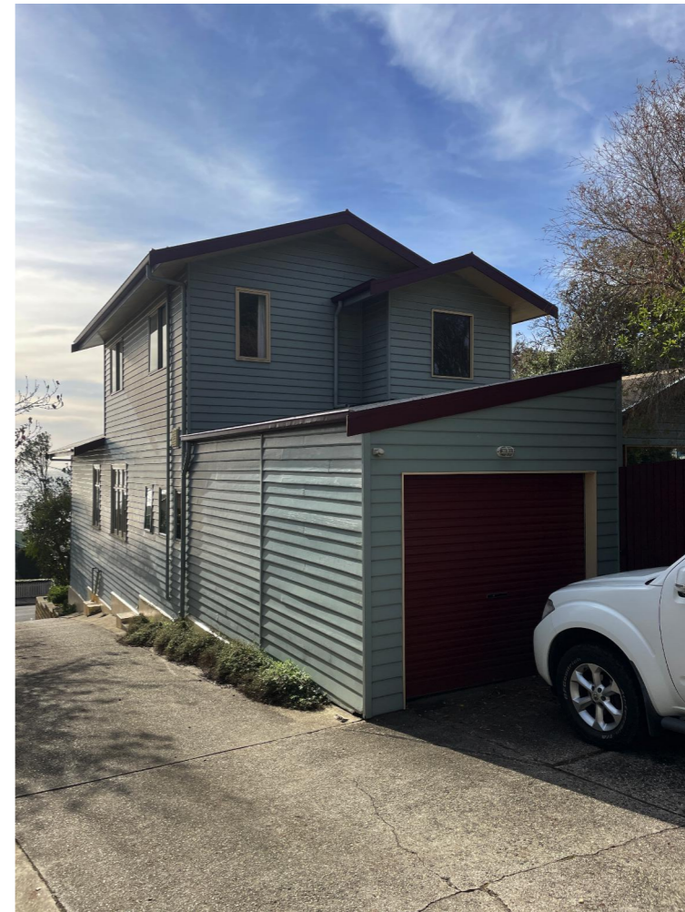
VIEW OF WEST FACADE FROM REAR
