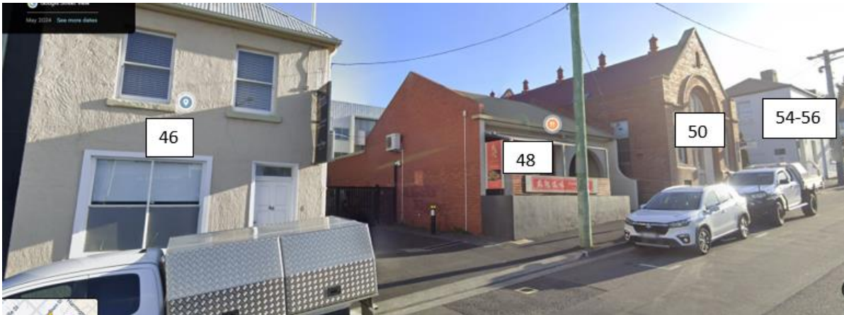
Figure 4: Travelling northwest up Barrack Street. The first on the left (46) is the Brow Studio and beauty / hair salon, then the laneway, the Yummy Inn City restaurant (48), the building used for emergency relief office and day shelter (50), 52 Barrack cannot be seen as it is set behind the building line. The double storey white building on the end is 54 and 56 Barrack housing the Hobart City Mission Op Shop.
