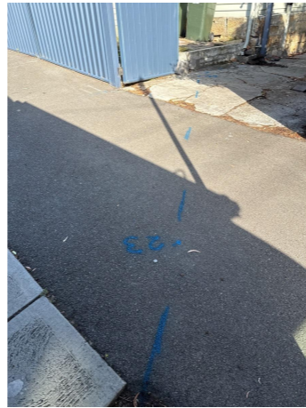
P2. STORMWATER LOCATED AT KERB CONNECTION
