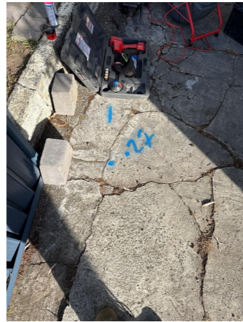
P1. STORMWATER BREAK IN PROPERTY
