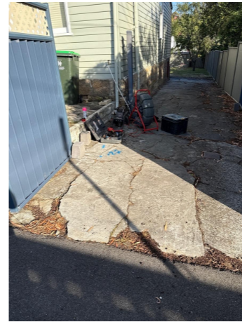
P3. STORMWATER PIT LOCATION
