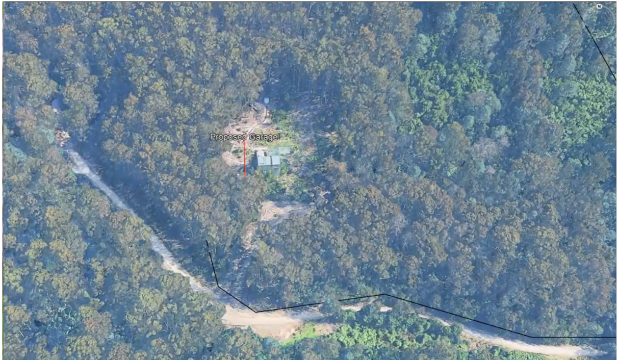
Looking from South
