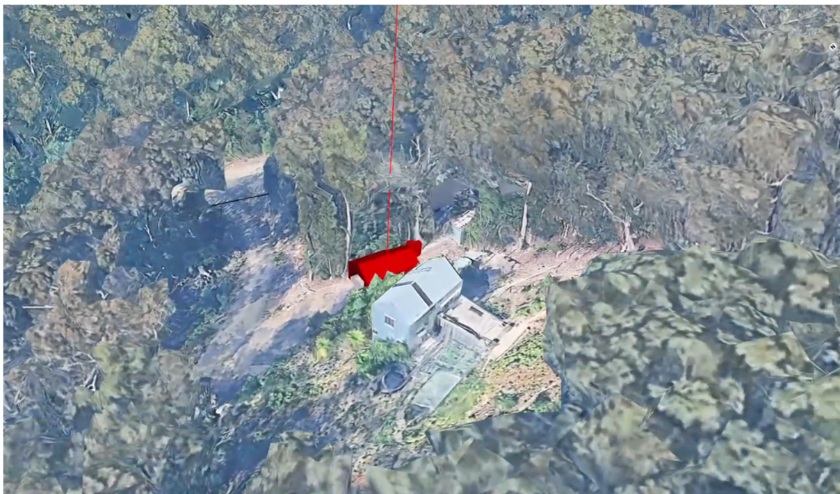
View showing shed nestled well out of sight behind vegetation.
