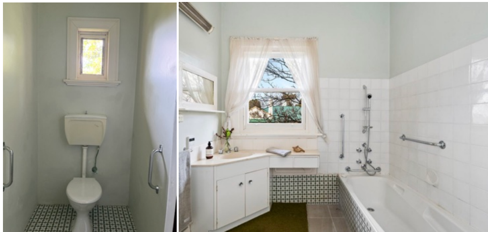
Demolition of non-original c.1950's wet area fittings and linings. Intrusive fabric.
