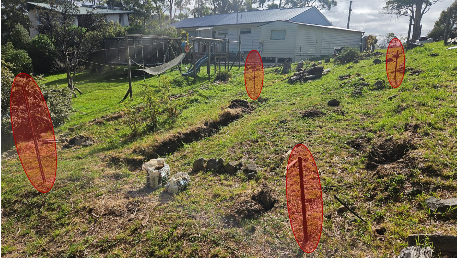
Existing vegetation is grass. Shed corner positions are shown by the highlighted red star pickets.
