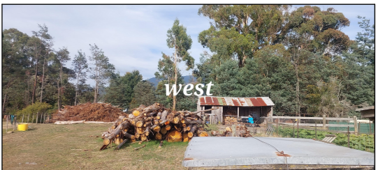
EXISTING ANIMAL ENCLOSURE IN STATE OF DISREPAIR TO BE DEMOLISHED. EXISTING WOOD SHED TO REMAIN.
