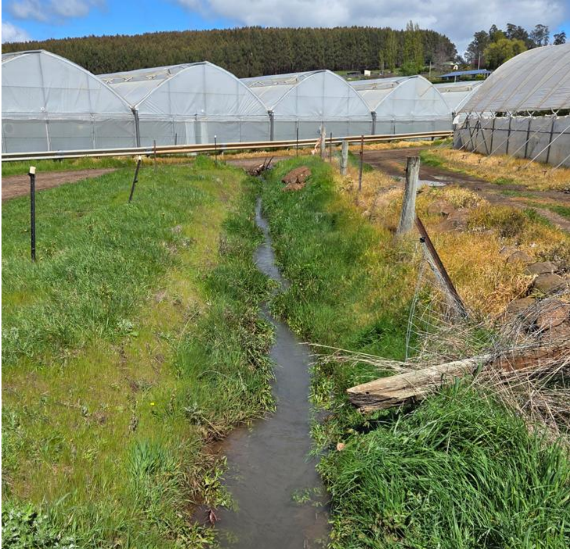
Figure 6 Northern drain typical construction through the site
