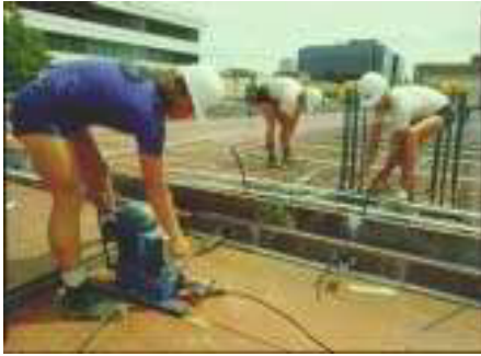
(a) Tendon placing
